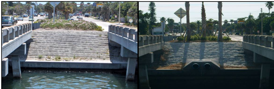
BEFORE AND AFTER OF DUEL PUMP STATION OUTFALL ON N BLVD OF THE PRESIDENTS BRIDGE TO MOTE MARINE
